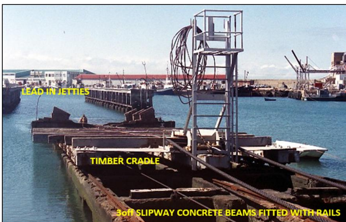
Figure 27: View from land to water showing slipway and jetties
