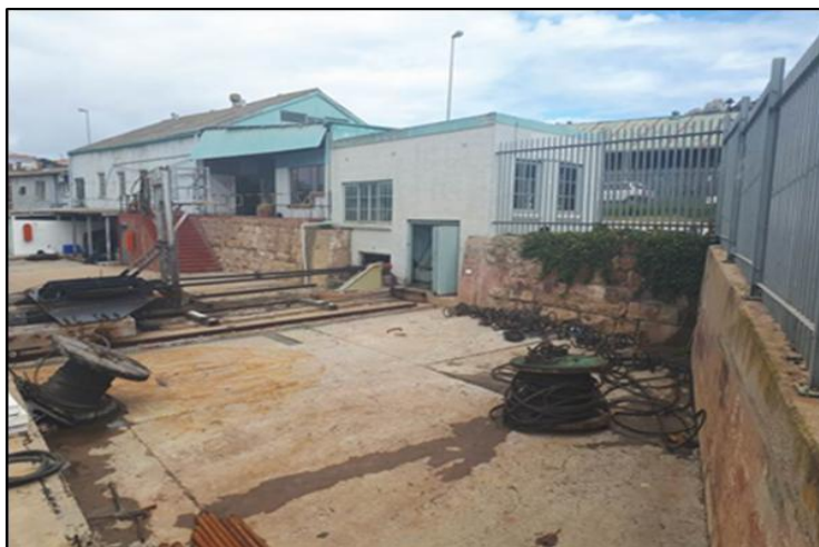
Figure 3: Slipway operations building
