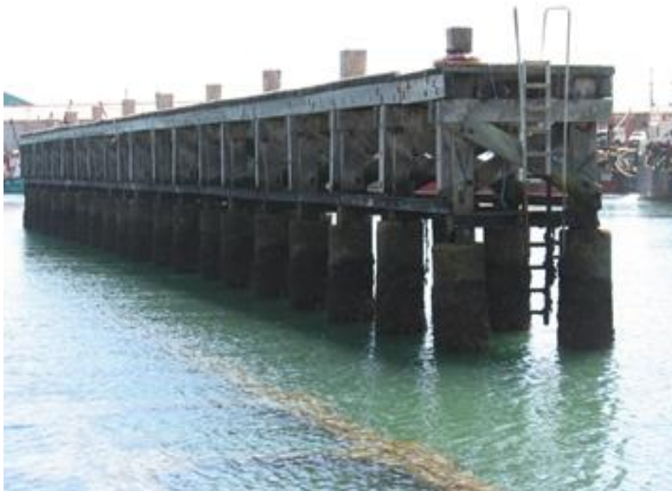
Figure 17: Existing lead-in jetties
